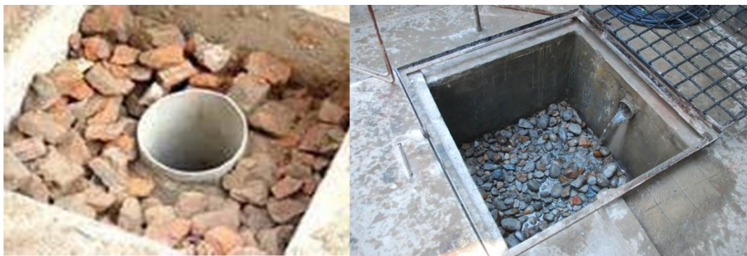
Recharge pits at Block 1 & Block2
